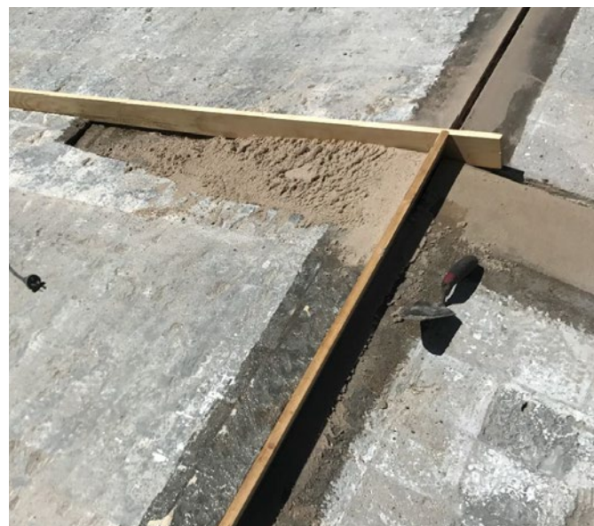
Epoxy resin system Repair to Joint Junction.
