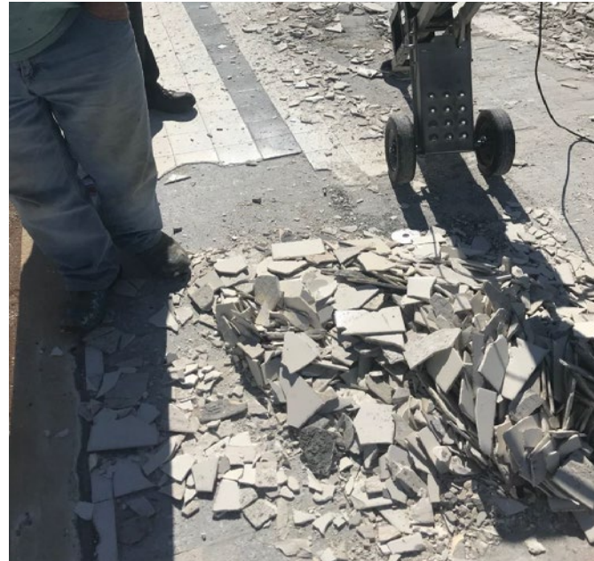
Removal of tiles and fiberglass lining.
