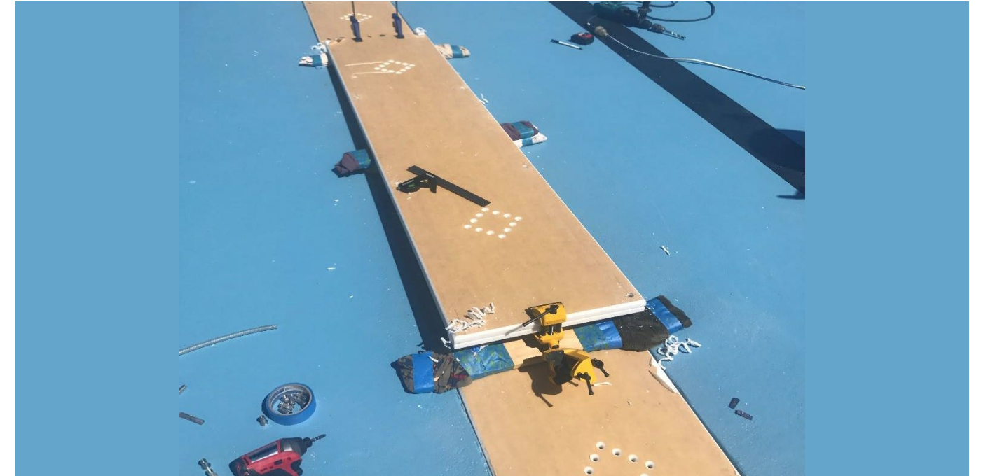
Installing and set up new centre feed line cover plates.
