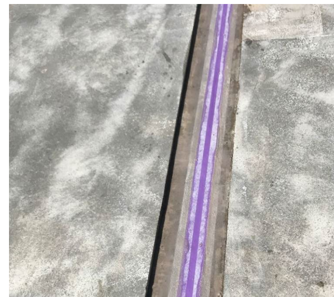
Joint band system installation to expansion joints.
