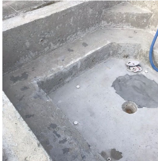
Removal of existing tiles
