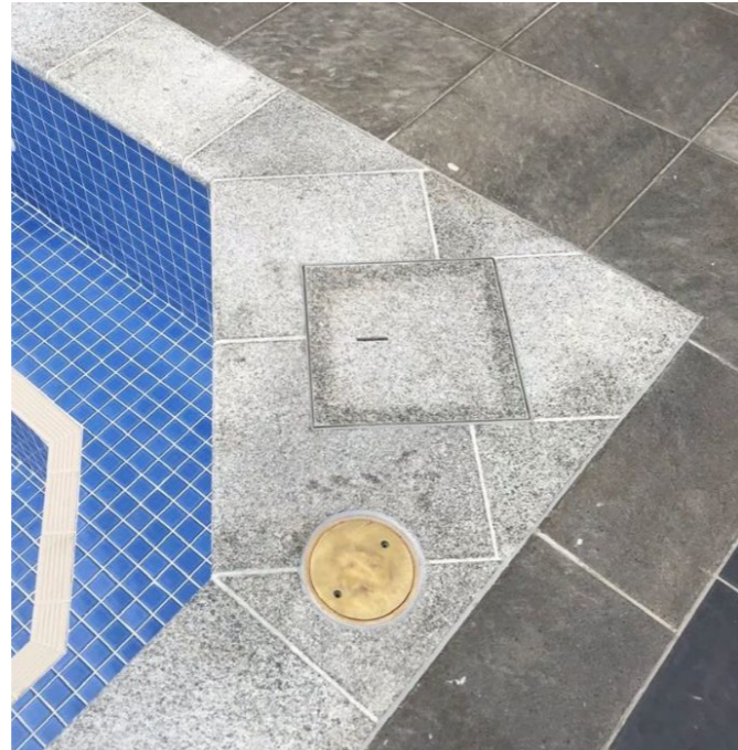
Tiling Spa - Skimmer box lid detail
