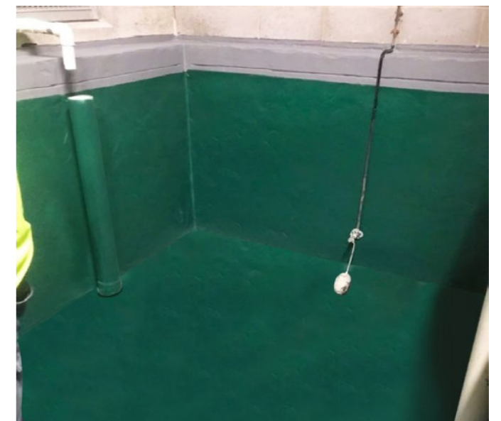
Sprayed Polyurethane membrane
