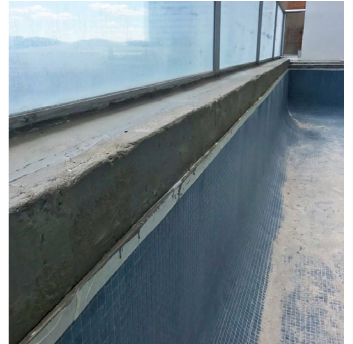
Waterproofing pool wet deck edge
