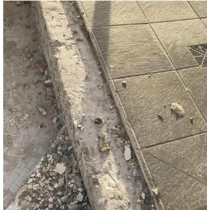
Removal of existing tiles
