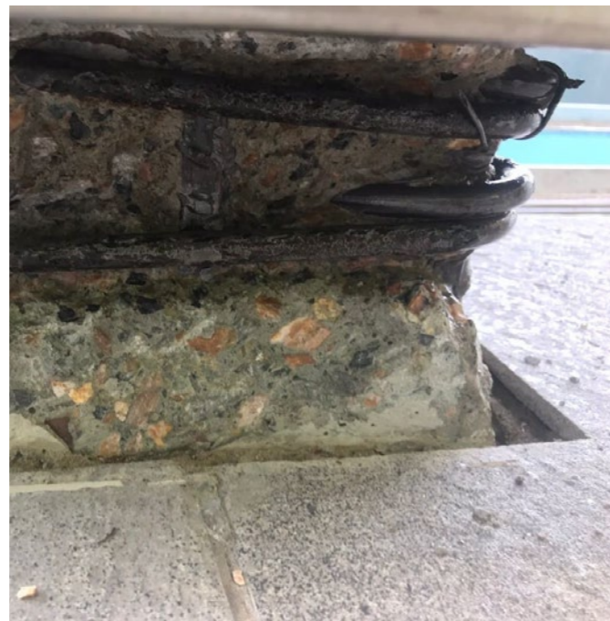
Remove spalling
