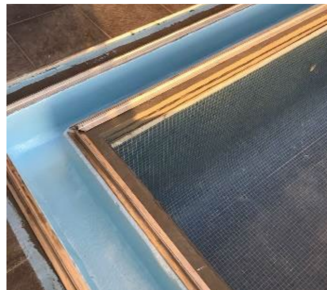
Epoxy Coating - Wet deck Channel
