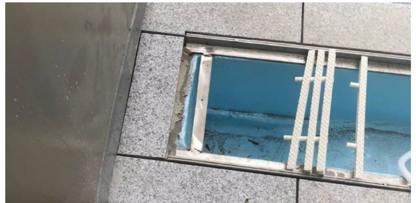
Tiling Wet Deck Concourse
