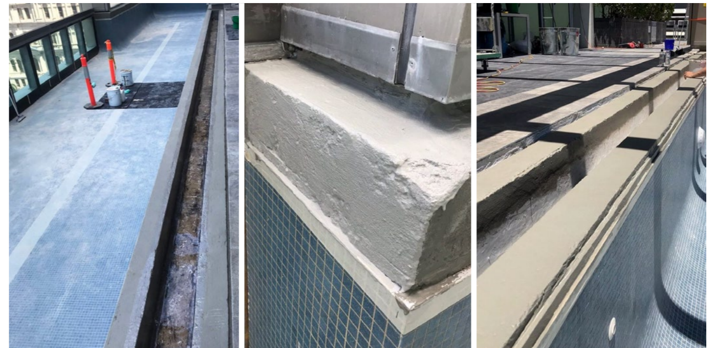
Completed waterproofing
