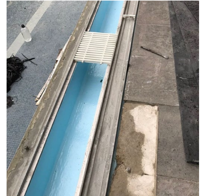
Stainless Steel installation - Wet deck Channel
