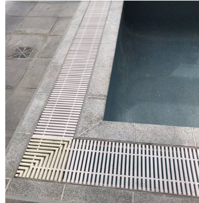
Wet deck grate re-installed
