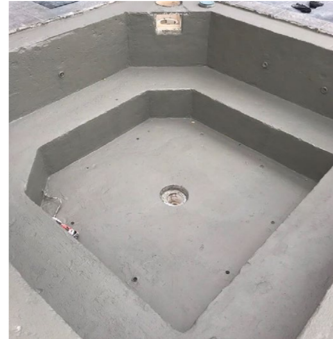
Waterproofing spa substrate
