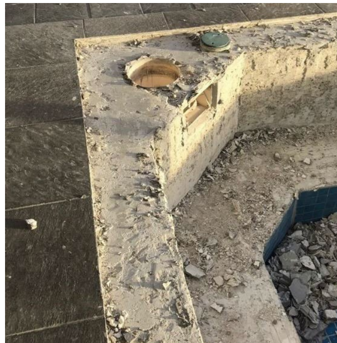
Removal of existing tiles
