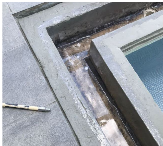
Waterproofing - Wet Deck Channel
