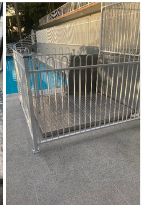
Pool Pump Pit Lid Refurbishment with new Aluminum Checker Plate Lid and matching fence
