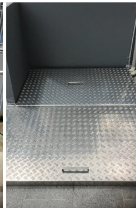
Pool Pump Pit Lid Refurbishment with new Aluminum Checker Plate Lid and matching fence
