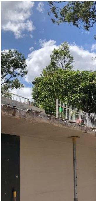
Excavate loose and flaky concrete
